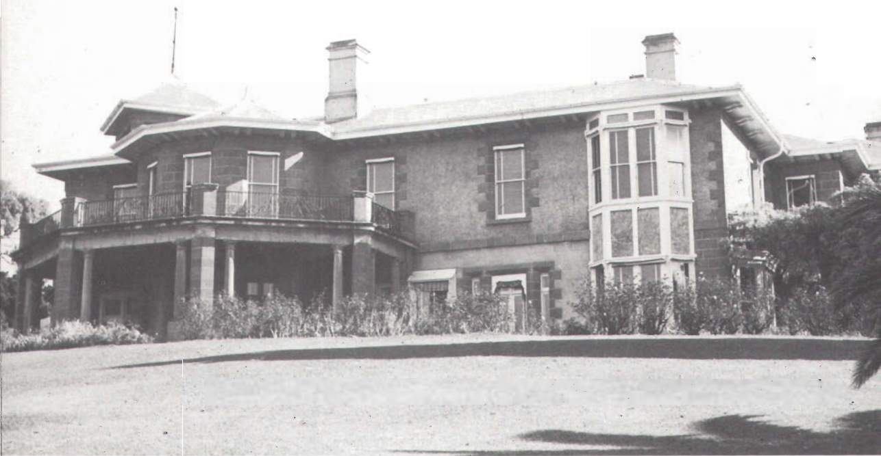
Glenormiston, near Terang. The old homestead is now used by the Agricultural College as its central administrative building.
